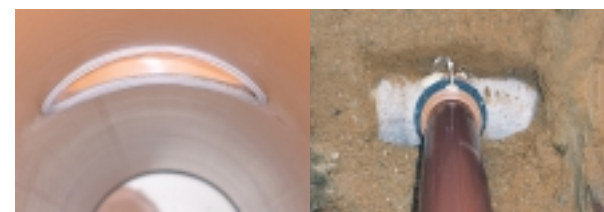
Correct installation of the junction.
